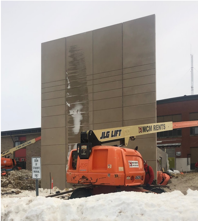
Larson works with Tri-State to stay ahead of the weather while setting the pre-cast walls. (photo by Cole Albaugh)
